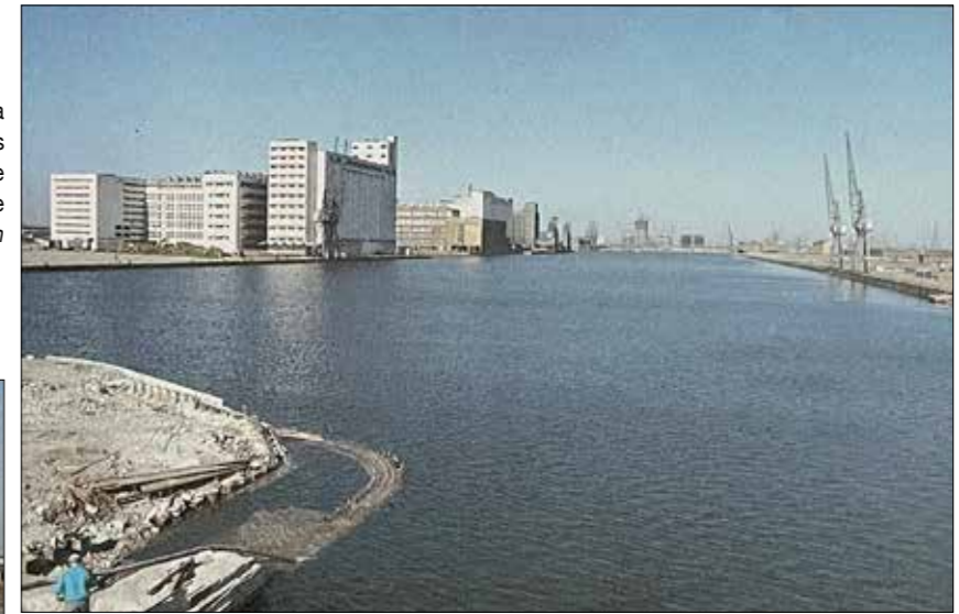
The vast Royal Victoria Dock (page 45) provides an impressive waterscape LEU/Ian Yarham
